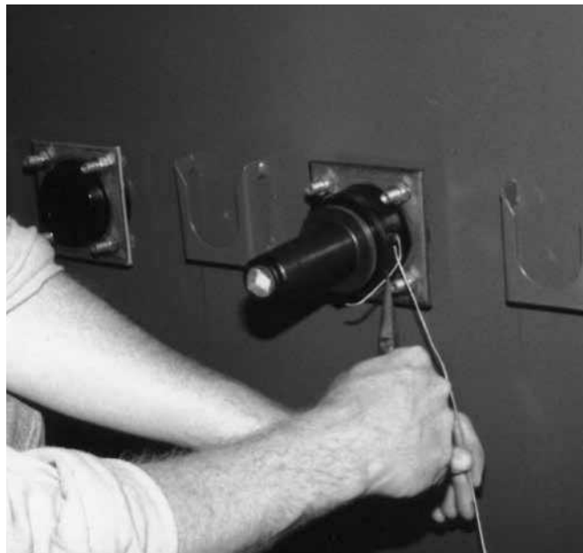
Figure 4. Attach ground lead (15 kV version shown).
